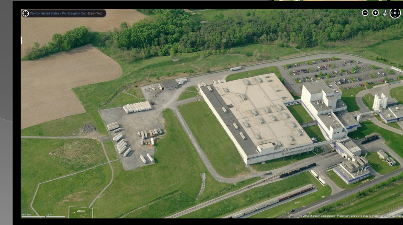
Plant before the expansion
